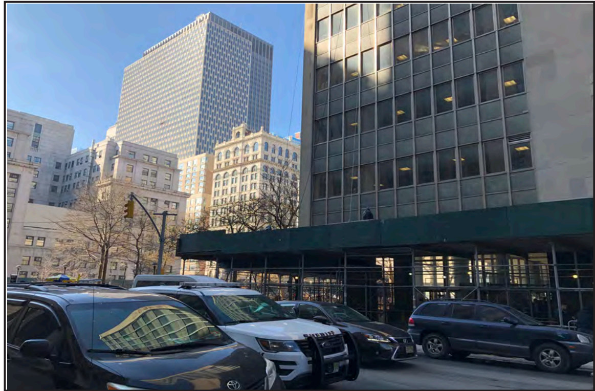
21) Looking southwest along Centre Street towards the Civil Court building.
