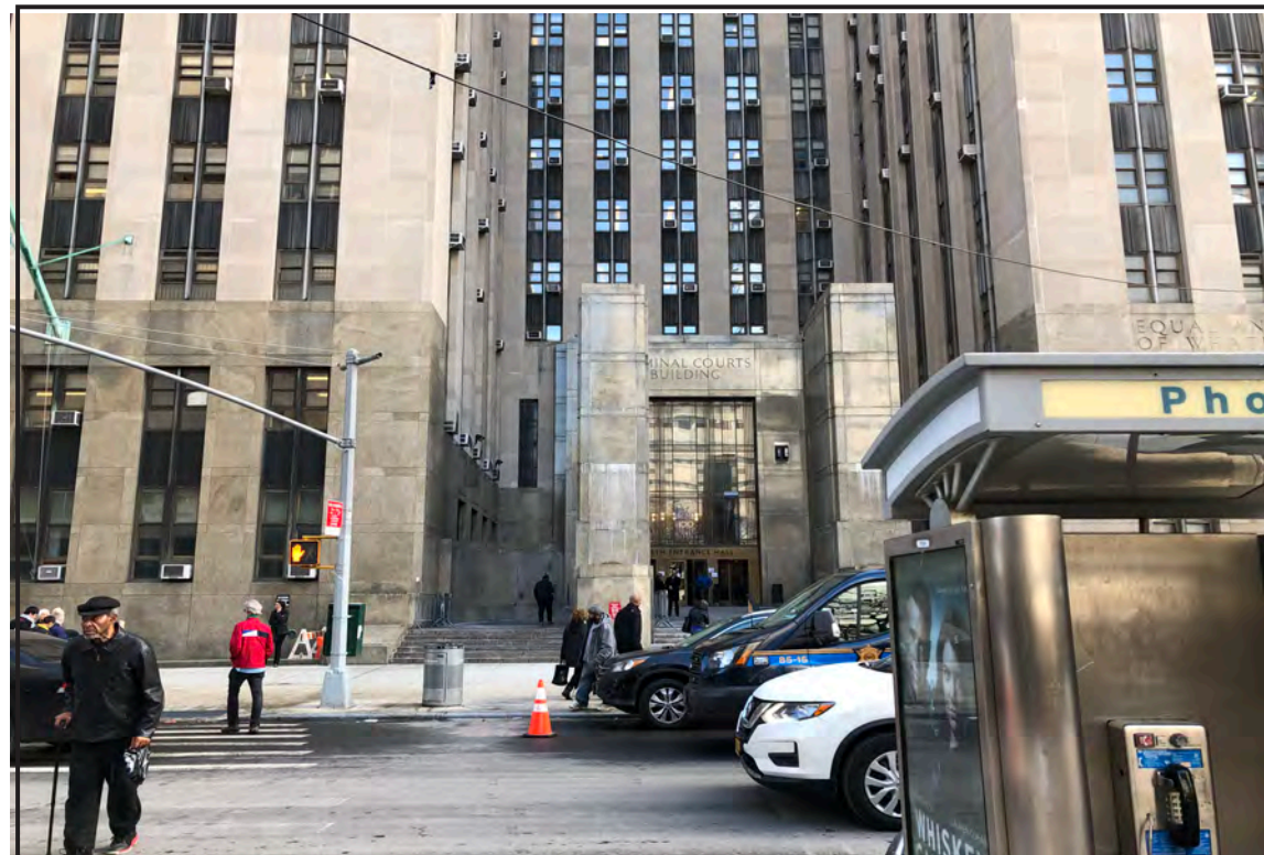
3) Looking at the southeast side of the criminal court building along Center street.
