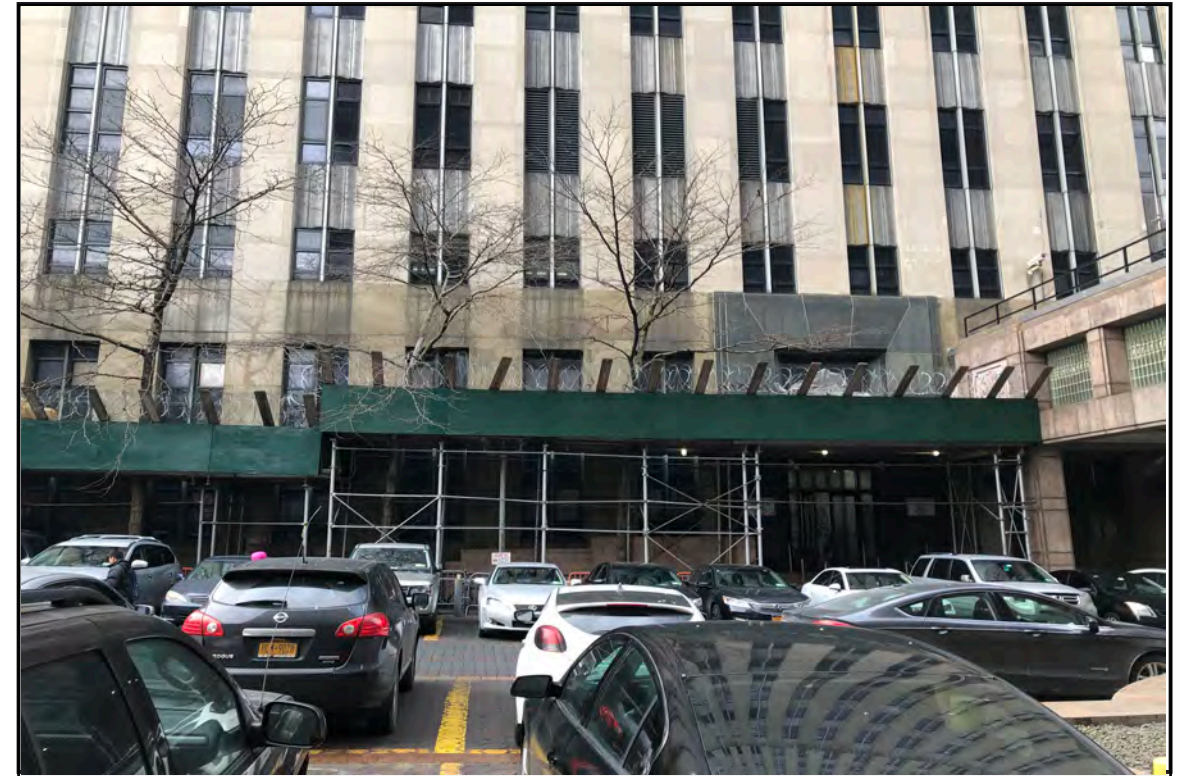
40) Looking south at the north end of the MDC South building, along White Street.
