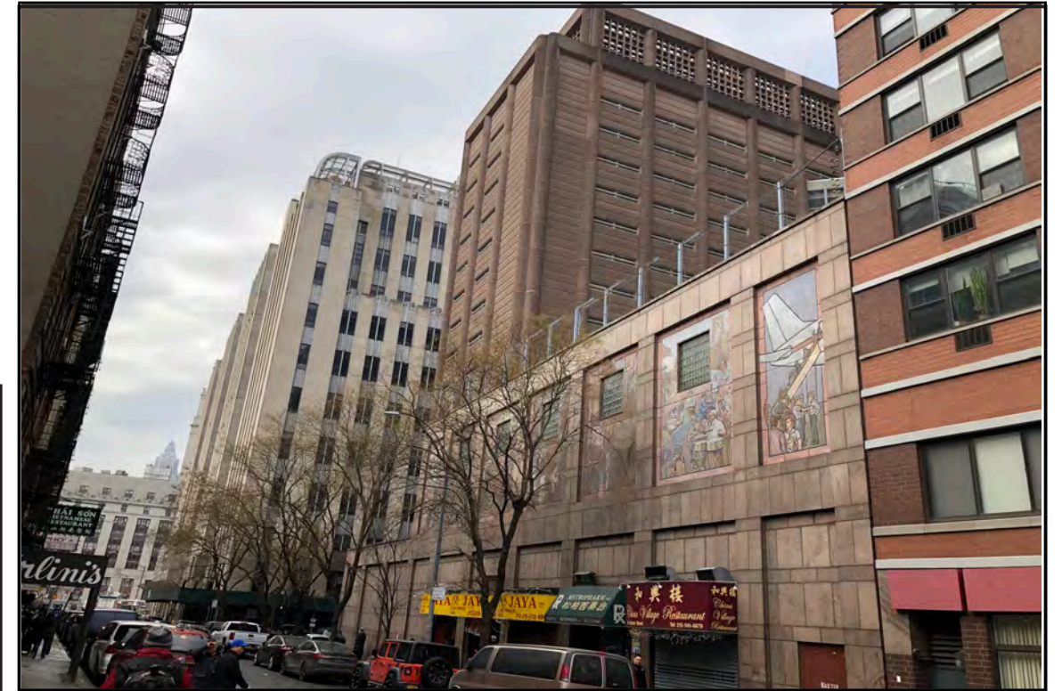
24) Looking southwest along Baxter Street; facing MDC North.
