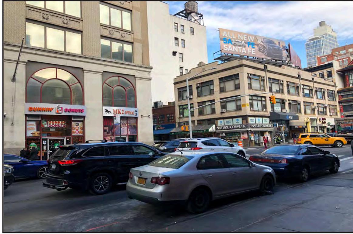
27) Looking northwest at the intersection of Walker Street and Centre Street.
