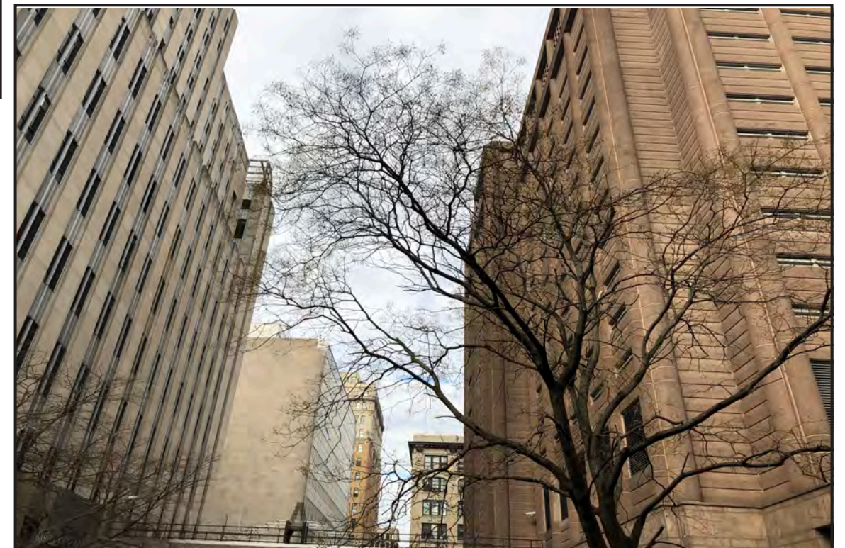
26) Looking northwest towards the southeast corner of the MDC North Building at the intersection of Baxter street and White Street.
