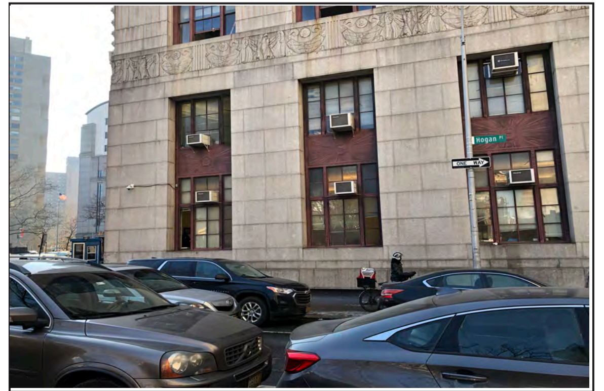
16) Looking southeast from the corner of Baxter Street and Hogan Place.
