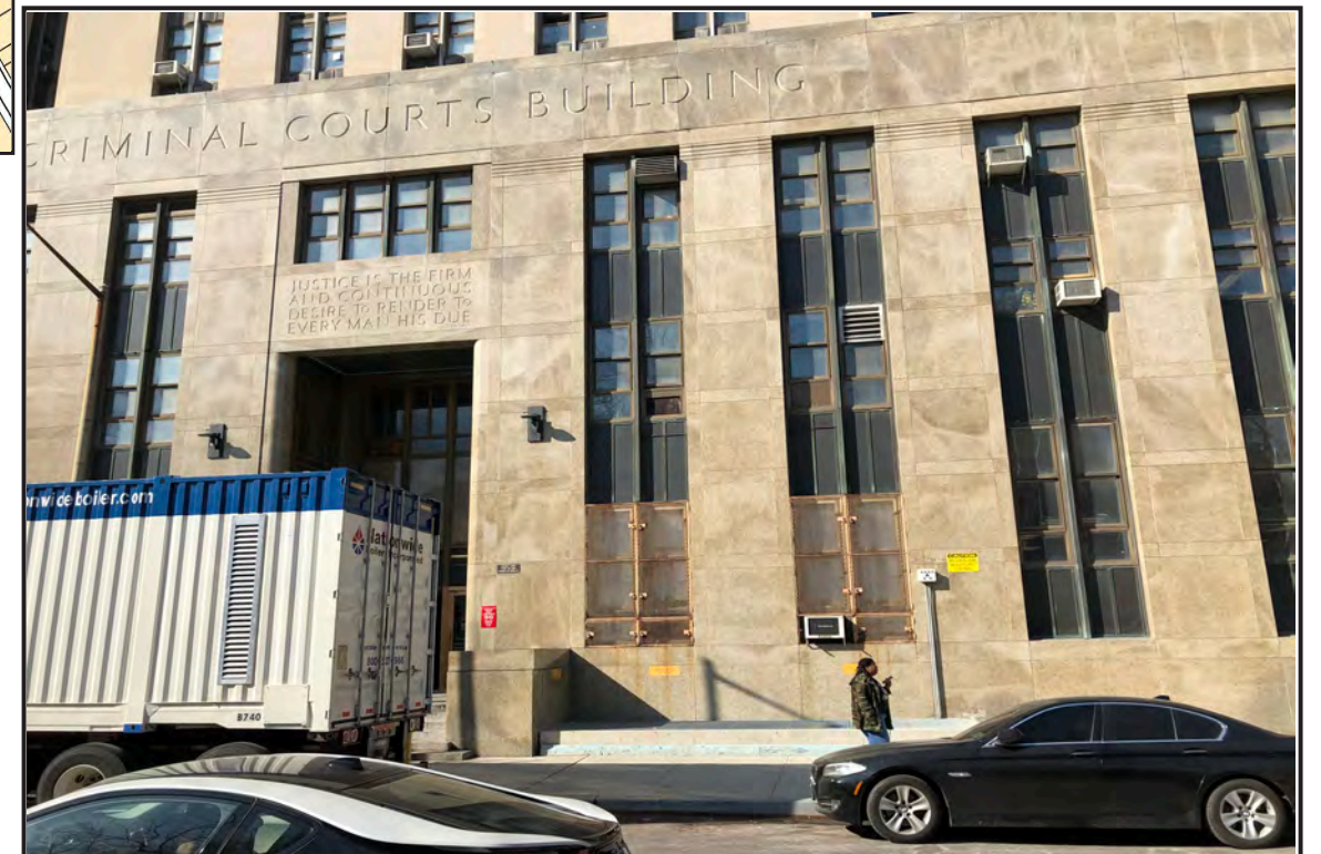
4) Looking at the southwest side of the criminal court building along Baxter street.
