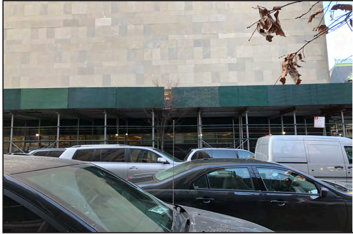
5) Looking at the northwest side of the civil court building along Center street.
